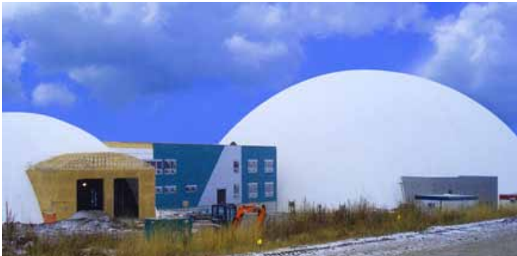
City of Edmonton Cloverbar Waste Management Center under construction
